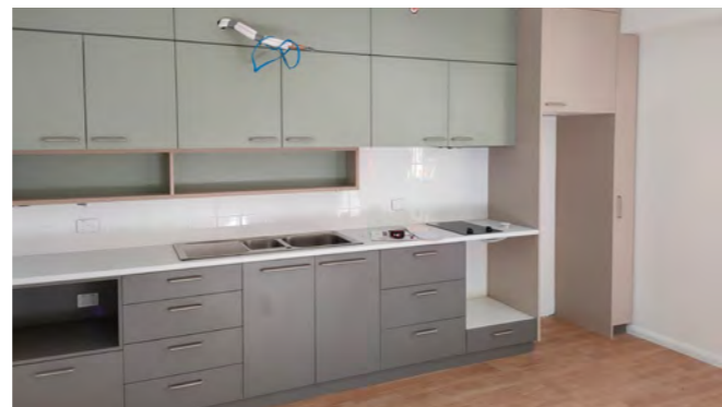
/ Internal fit-outs at Lyndell White House are coming along nicely.
