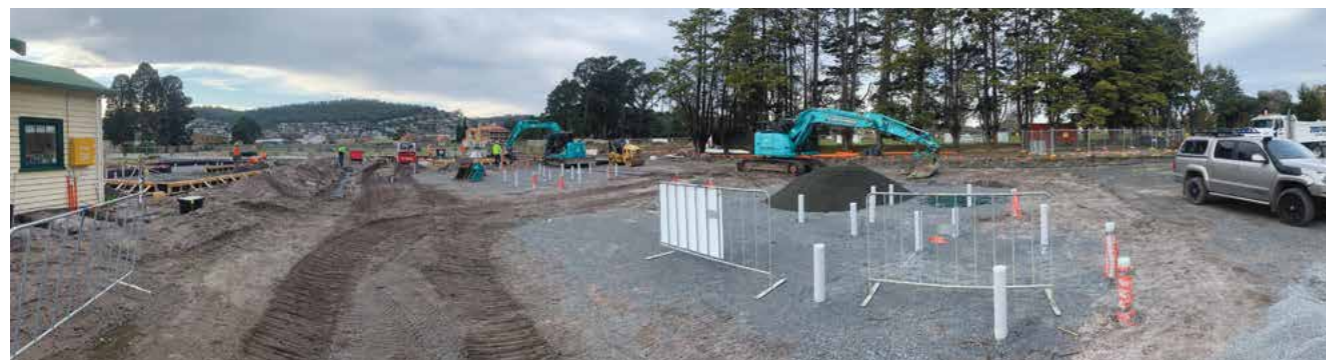
Construction is underway in Tasmania.
